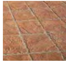
Stamped Concrete Paving (Bomanite, Rustic Slate)
