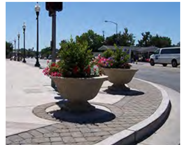
Bulbouts/ curb extensions are recommended at all crossing areas for pedestrian amenities to reduce crossing distances, slow traffic, and allow for driver awareness of pedestrians.
