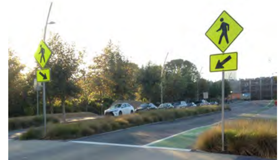
Example of pedestrian crossing signage being used to alert vehicles of the crosswalk.
