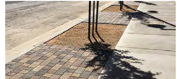
Unique and recognizable paving materials should be utilized at streetscape furnishing and edge zones
