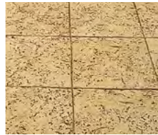
Stamped Concrete Paving (Bomanite, Coquina)
