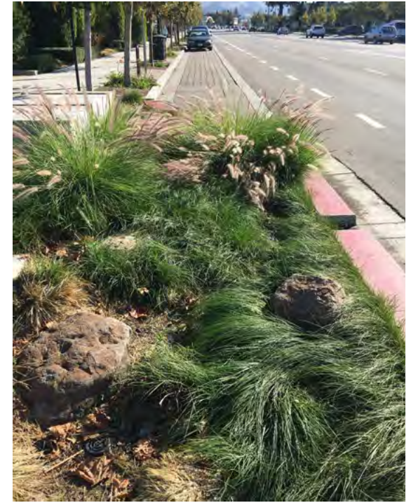
Storm water planting areas should provide year-round interest and thrive in wet and dry conditions.
