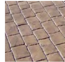
Stamped Concrete Paving (Bomanite, Used Brick)
