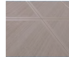
Broom Finish Concrete
