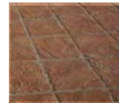
Stamped Concrete Paving (Bomanite, Rustic Slate)
