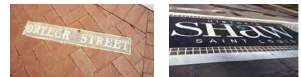
Examples of paving insets in sidewalks and/or crosswalks to aid in pedestrian wayfinding
