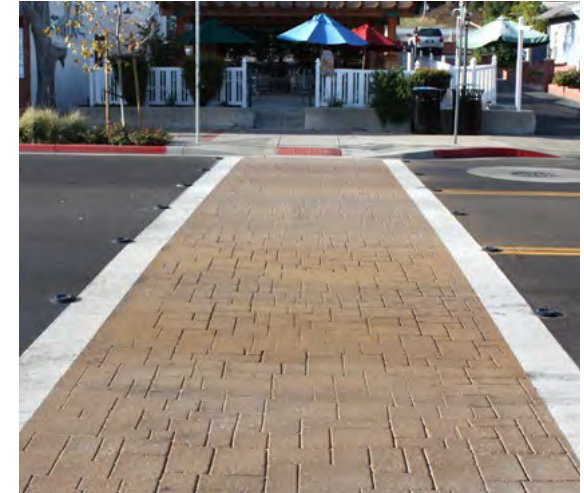
Example of a crosswalk with stamped asphalt paving in a ashlar slate pattern
