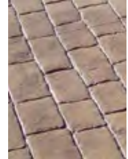
Example of Edge Zone Decorative Paving: Stamped Concrete Paving (Bomanite, Used Brick)
