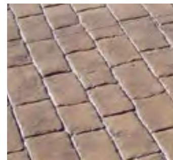
Example of Furnishing Zone Decorative Paving: Stamped Concrete Paving (Bomanite, Used Brick)
