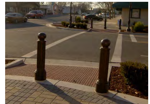
Decorative bollards are recommended at primary intersections to visually designate crossing areas
