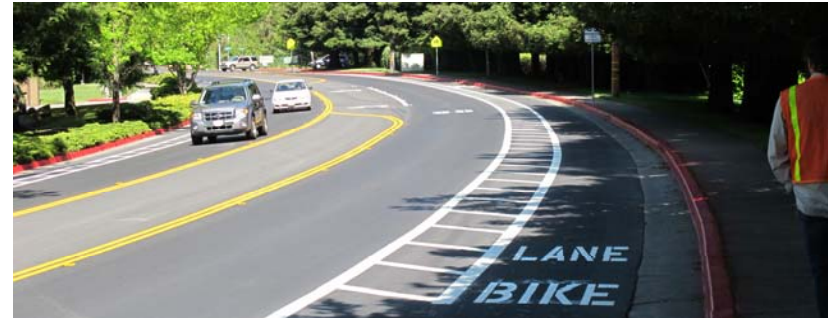
A typical buffered bicycle lane
