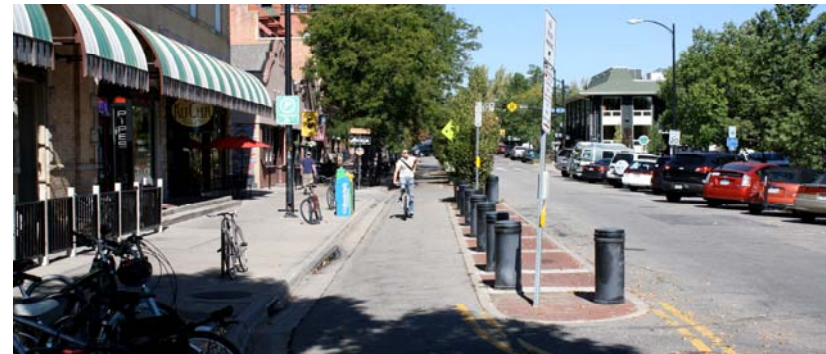
Typical separated bikeway with bollards
