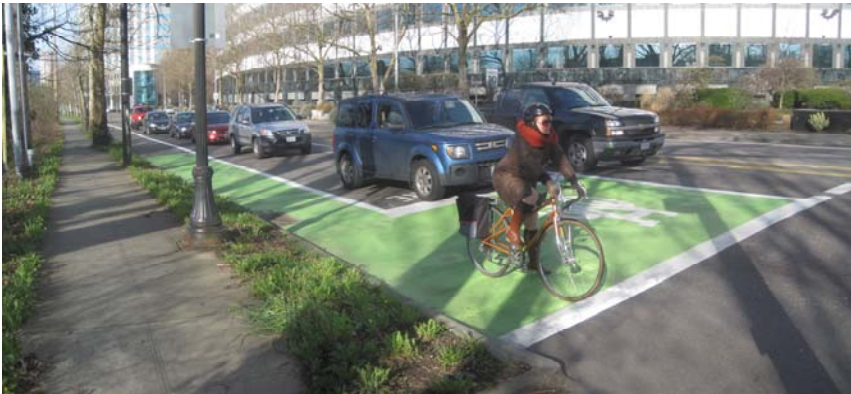
Typical bicycle box
