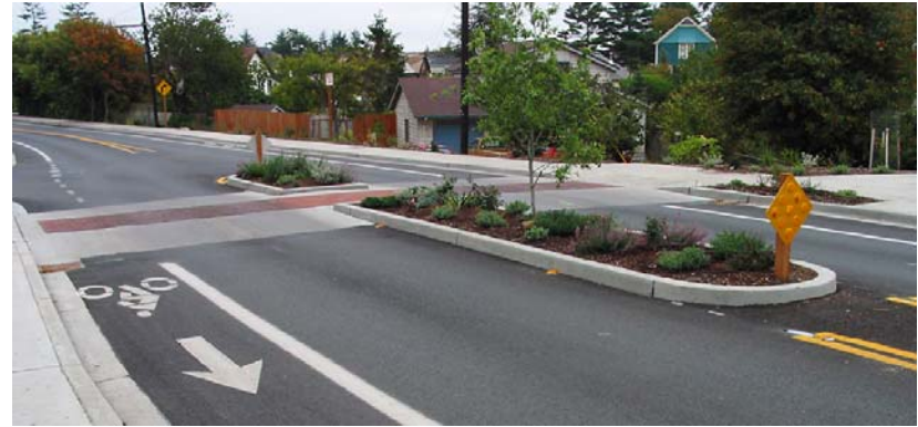
A typical median refuge
